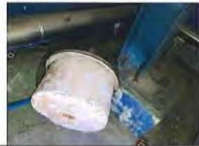
Reversing chamber - smoke tube 2 nd pass
