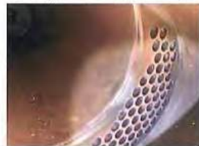
Reversing chamber - back end
