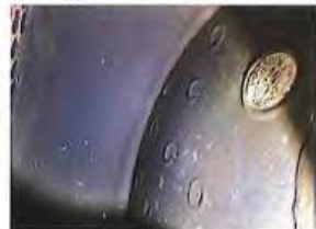
Rear end plate - smoke tube 3 rd pass
