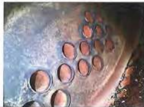
Rear end plate - smoke tube 3 rd pass
