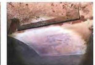
Reversing chamber - Flame tube / wet back
